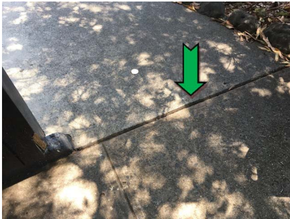
Photo 3. Exterior, north elevation, throughout pavement, expansion joint – non asbestos-containing construction mastic.
