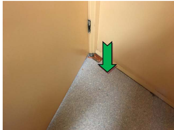
Photo 4. Interior, work room, light blue floor coverings – non asbestos-containing vinyl sheet.
